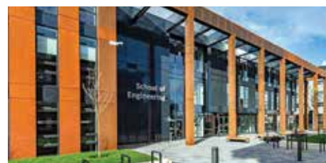
The University of the West of England's NEC4-procured Engineering Building won overall Project of the Year
