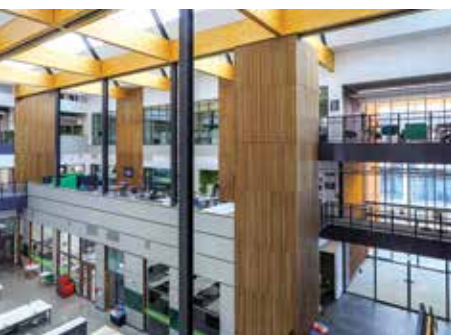
The 8500 m 2 building's full-height atrium is finished with a glulam timber roof structure
