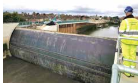
The Environment Agency's ongoing ECC Boston Barrier scheme won Climate Resilience Project of the Year
