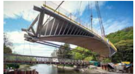
The 40 m long, 300 t stainless-steel and concrete composite structure was installed in a single lift
