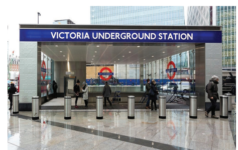
The NEC-procured upgrade doubled the size of Victoria Underground Station in central London, including a new north ticket hall
