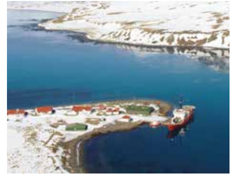
▲ NEC3 TSC is being used to extend the existing wharf at King Edward Point environmental research station in South Georgia
